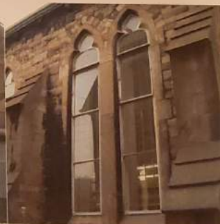
Cast-iron fixed frame windows.
