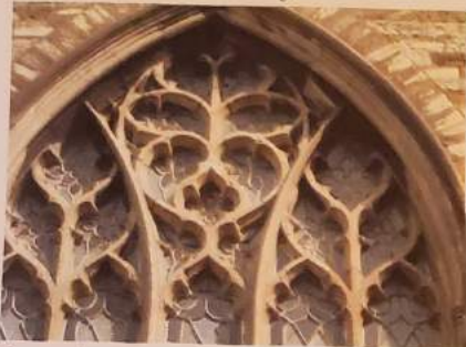
Carved stone window detailing
