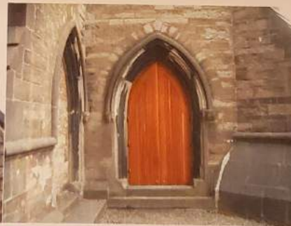
Arched wooden double door. Doors to south + east elevation now blocked up.
